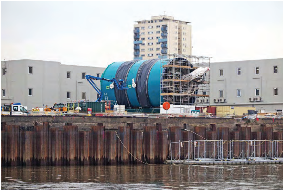
Tunnel boring machine assembly, Kirtling Street
